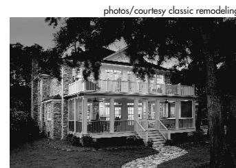
The house was extended 20 feet to the rear and a two-story porch was added that offers panoramic lake views from both levels. The upper porch is accessed through French doors from a new second-story master suite with wings at either end. Downstairs, an open floor plan enables the centrally located kitchen to meld with the family room, which is accented by a coffered ceiling and two-sided hearth that also serves the adjacent library.
